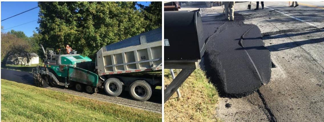
Fig. 5.5. Field view of overlay on Cropper School Road in Pleasureville, KY
