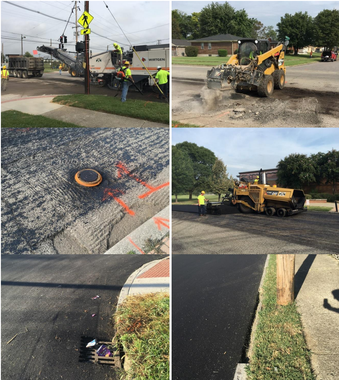
Fig. 5.7. Field view of mill and overlay on Southern Avenue in Louisville, KY
