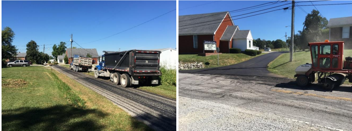
Fig. 5.6. Field view of overlay on Flood Road in Pleasureville, KY
